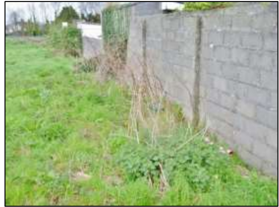
JK 1 : South eastern boundary wall, looking east – March 2019
