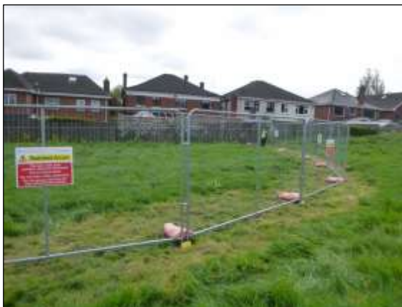
JK 1 : Fitting temporary fencing and advisory signage - May 2019
